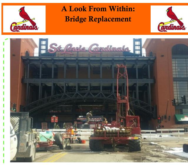
We wanted to highlight this recent project because of the location of the site. This project required soil borings that included split-spoon sampling, Shelby tubes and rock coring for a bridge replacement over the Metro-Link tracks just west of Busch Stadium. The two borings were drilled by our experienced crew that consisted of Chad Dutton & Charlie Jones. One of the borings was completed as a flush mount monitoring well and the other was grouted closed with cement/bentonite grout.
